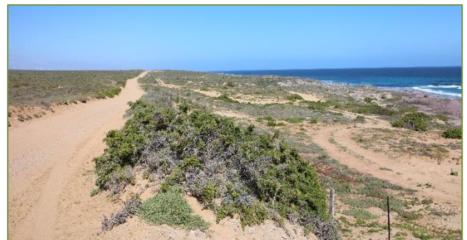
Figure 2: Existing gravel roads will require upgrading
